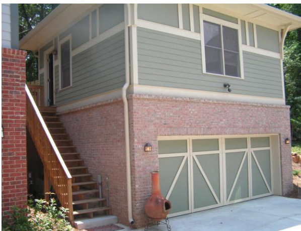
Accessory Dwelling Units in new urban community (Glenwood Park); accessory apartments are built above the garage and constructed along with the primary dwelling. Architecture and design elements of each ADU match those elements of the main dwelling.
